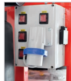
Single phase with 3 motors plus 1 filter shaker motor
